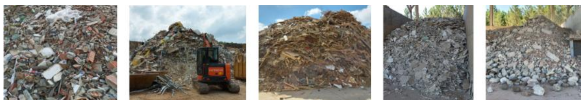
Figure 4. Separation of CDW by type (a) CDW requiring separation (b) Ongoing separation (c) Wood waste (d) Plasterboard waste (e) CDW—suitable (Pacheco & de Brito, 2021).
